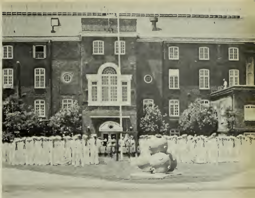
OLD TIMER —When Mine Force moved from Norfolk in 1946 it established its headquarters in this building. Below: USS Bluebird (MSC 121) heads to sea.
